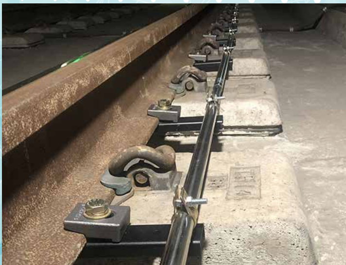
Monitoring for railways | Concrete roadbed
