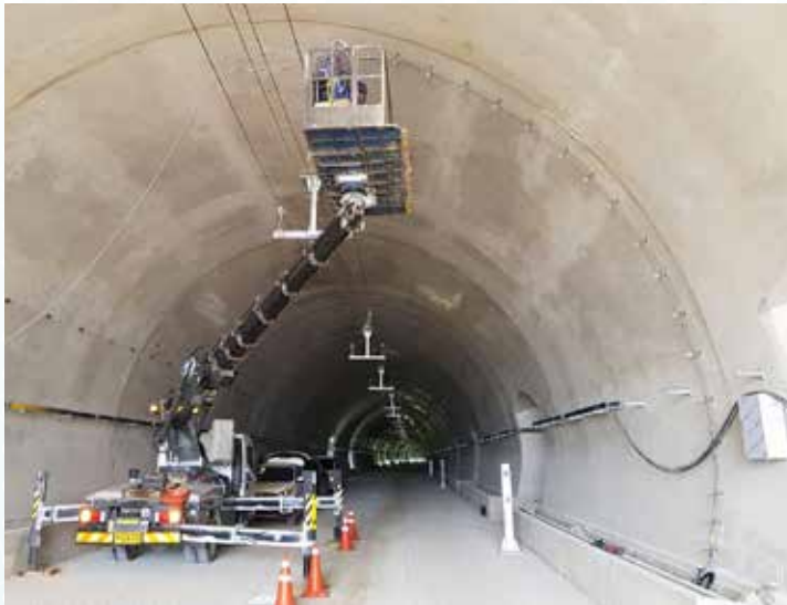
Convergence measurement of tunnel
