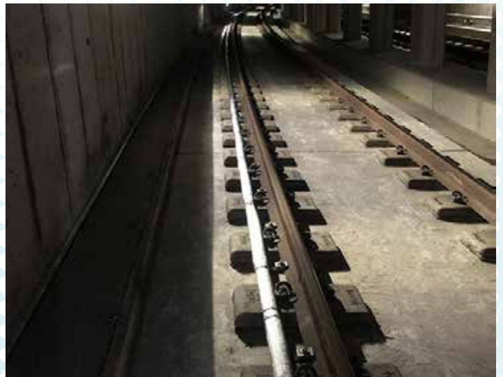
Monitoring for railways | Concrete roadbed
